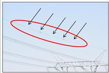
Figure 5: Some bird-diverters have been installed.
